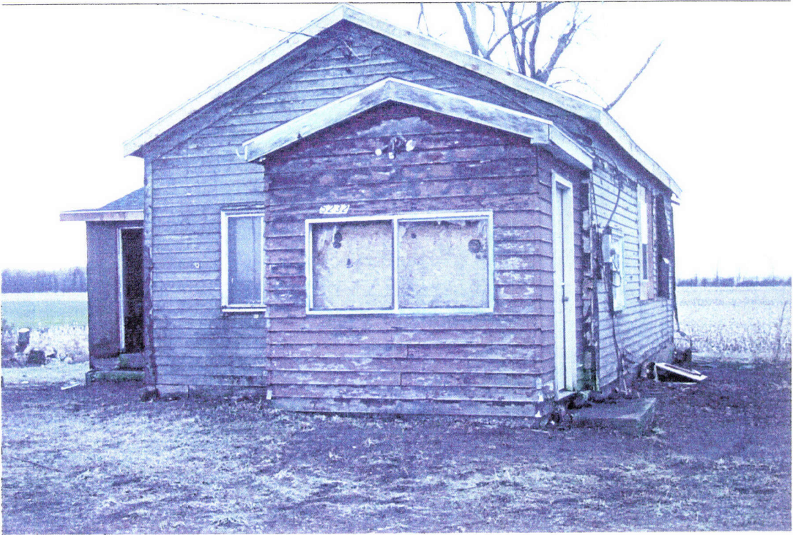
Photograph 13 5232 South Woods Road Looking Northwest
