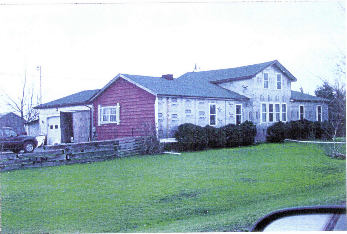
Photograph 14 5317 South Woods Road Looking South
