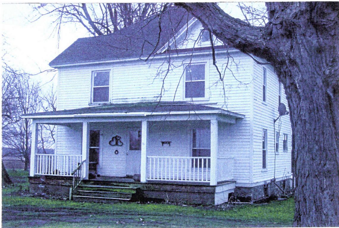
Photograph 6 Unmarked Residence (Fletcher Chapel Road) Looking Southeast
