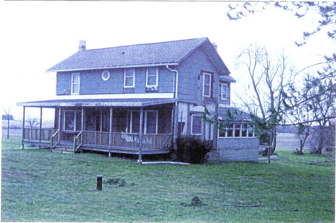
Photograph 12 12016 Fletcher Chapel Road Looking Southeast
