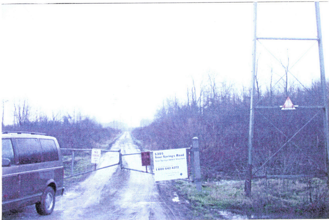
Photograph 22 Driveway for Substation (Sour Springs Road) Looking West
