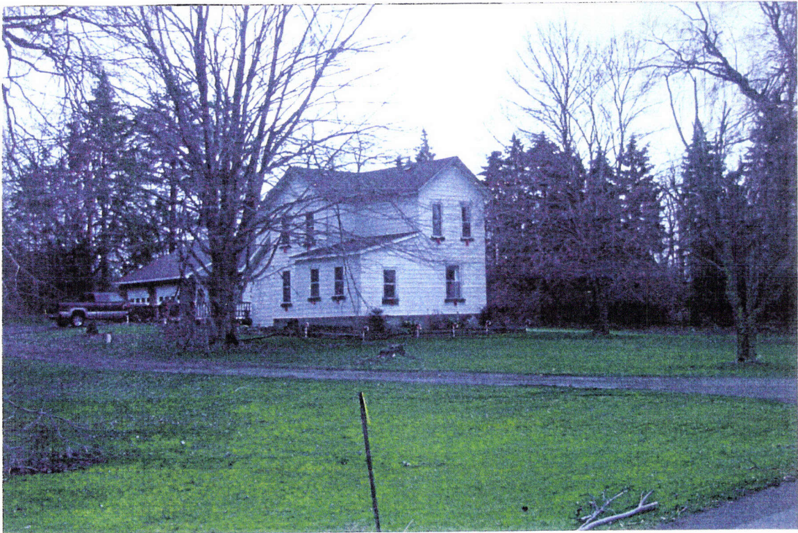
Photograph 8 Unmarked Residence (Fletcher Chapel Road) Looking North
