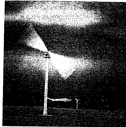
Siting wind farms far from avian flight paths can greatly reduce bird kills; taller turbines with fewer arms also help.
